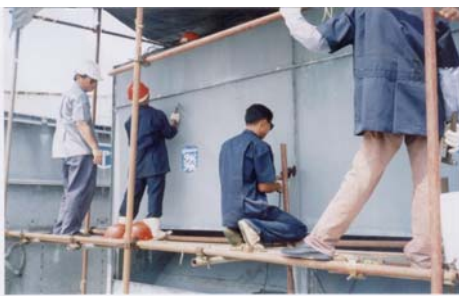
Install scaffolding on both sides
