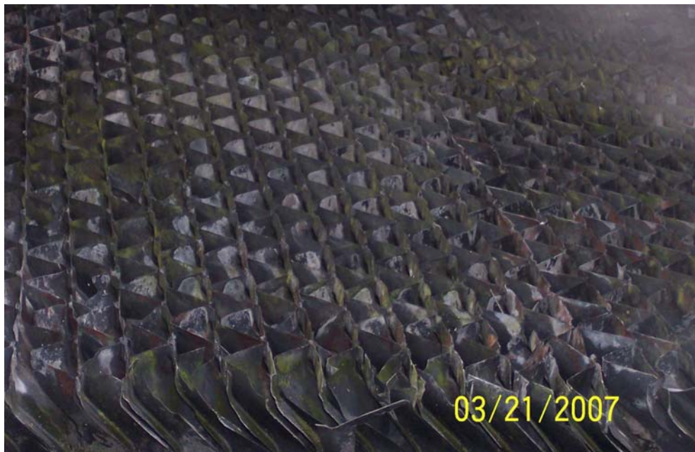
Top-side drift screens on day 41 of the evaluation, cleaned and scale-free due to Micro-Nice® D-5's action through tower sprays with no hosing or power-washing.
